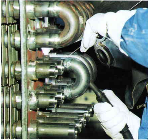
Prefabrication of economizer section
